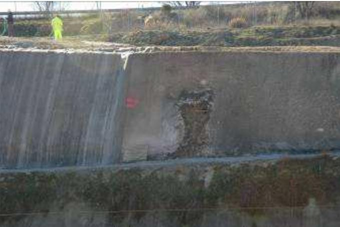
Figure 16. Appearance of the gunita next to MdH. The gunita burst due to the ground water.
