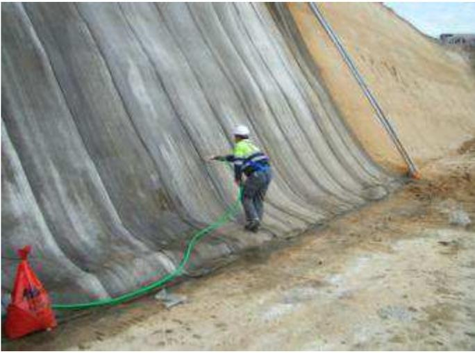
Figure 15. MdH hydration by water spread.
