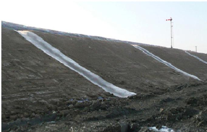
figure 32. CC5 was specified to build several down ditch linings.
