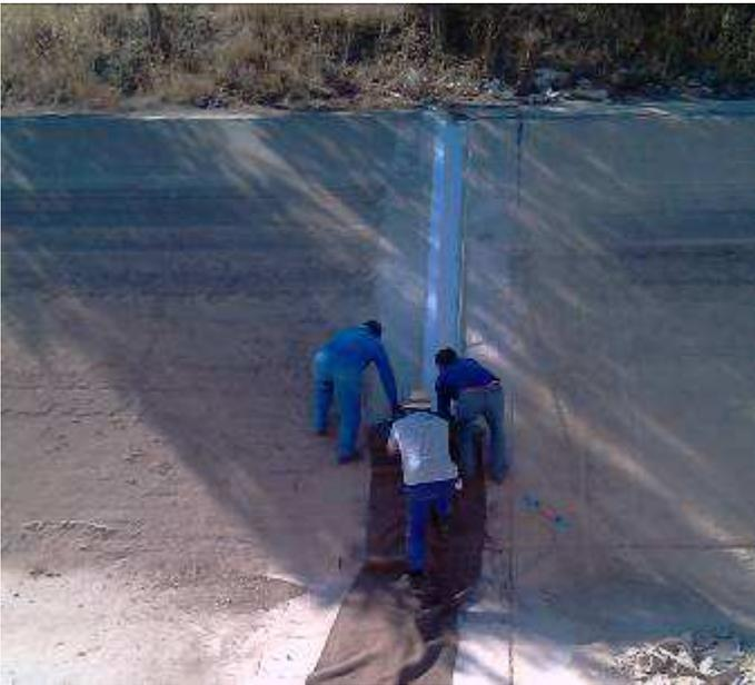
Figure 19. Placement of MdH on the joint.
