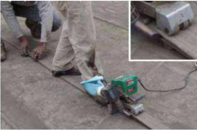
Figure 25. automatic thermal welding procedure.
