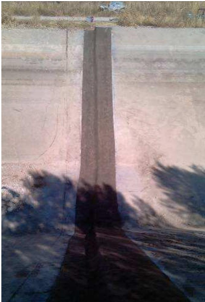
Figure 20. Appearance of the joint repaired
