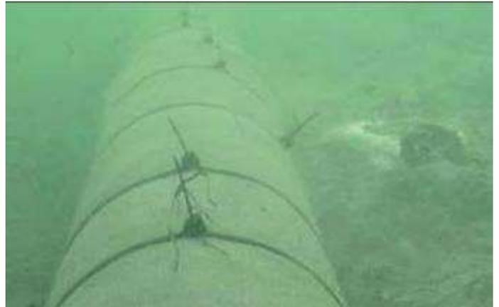
Figure 37. Pipe protection made with MdH under sea water.
