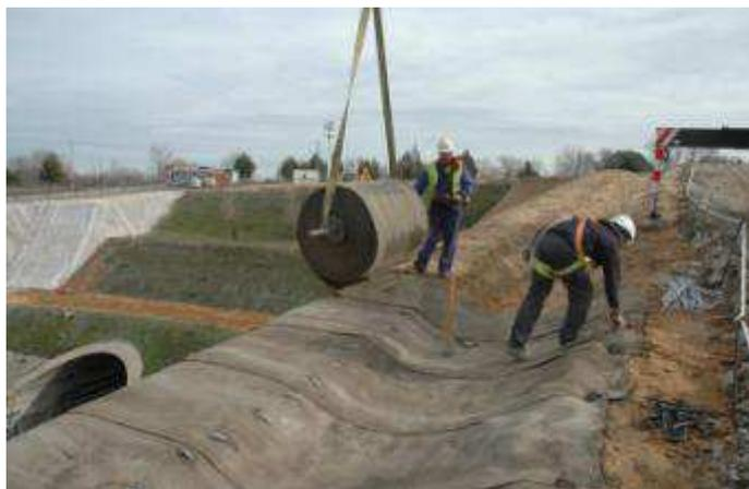
Figure 14. Continuous surfacing from the ditch lining in the top to the toe of slope.
