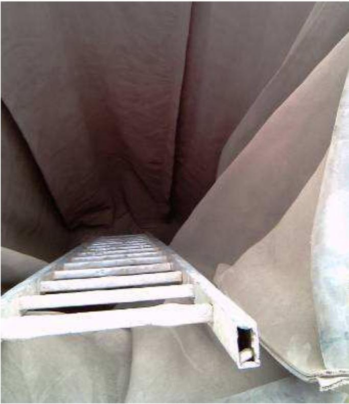
Figure 36. Tailored canvas placed inside the siphon before being hydrated.
