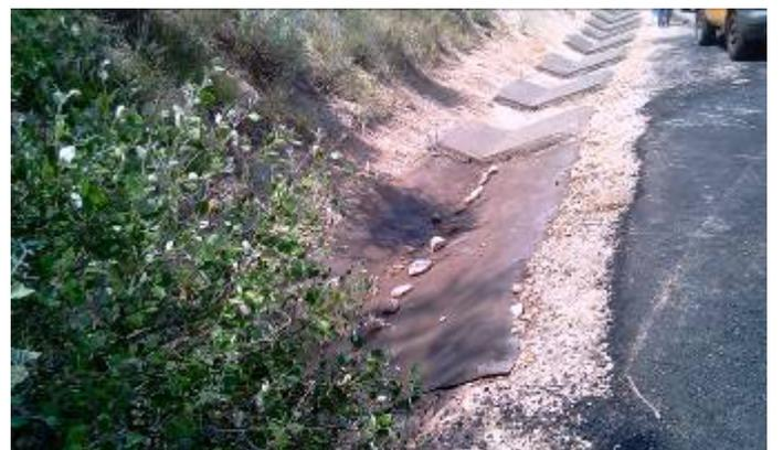
Figure 30. MdH ditch next to a conventional ditch
