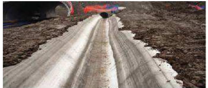
Figure 4. Ditch lining.
