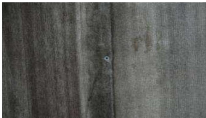
Figure 13. Steel screws were used to attach adjacent layers.
