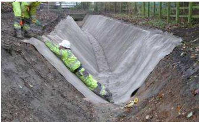
Figure 33. Deep ditch lined with MdH.
