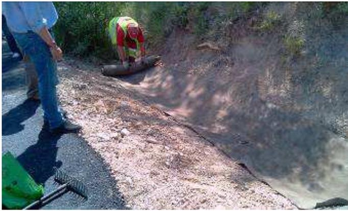
Figure 31. Ditch lining with MdH.
