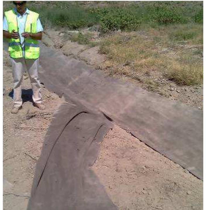
Figure 28. Ditch lining.
